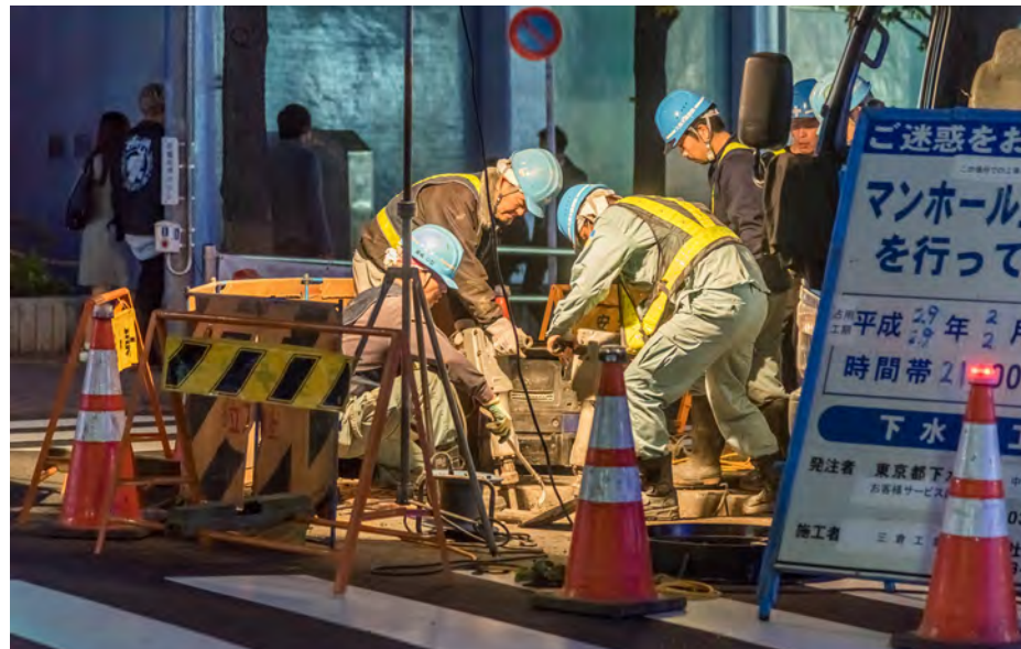
Underground utility repair in Tokyo's Shibuya ward
